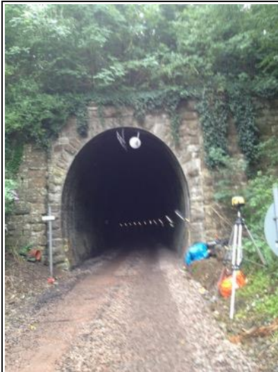
Photo 15. Railway tunnel (Pill) Date: November 2016
