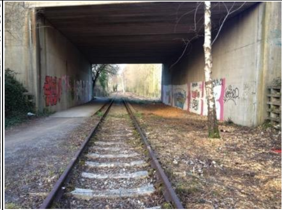
Photo 2. Bridge 4 with bat roost Date: August 2015
