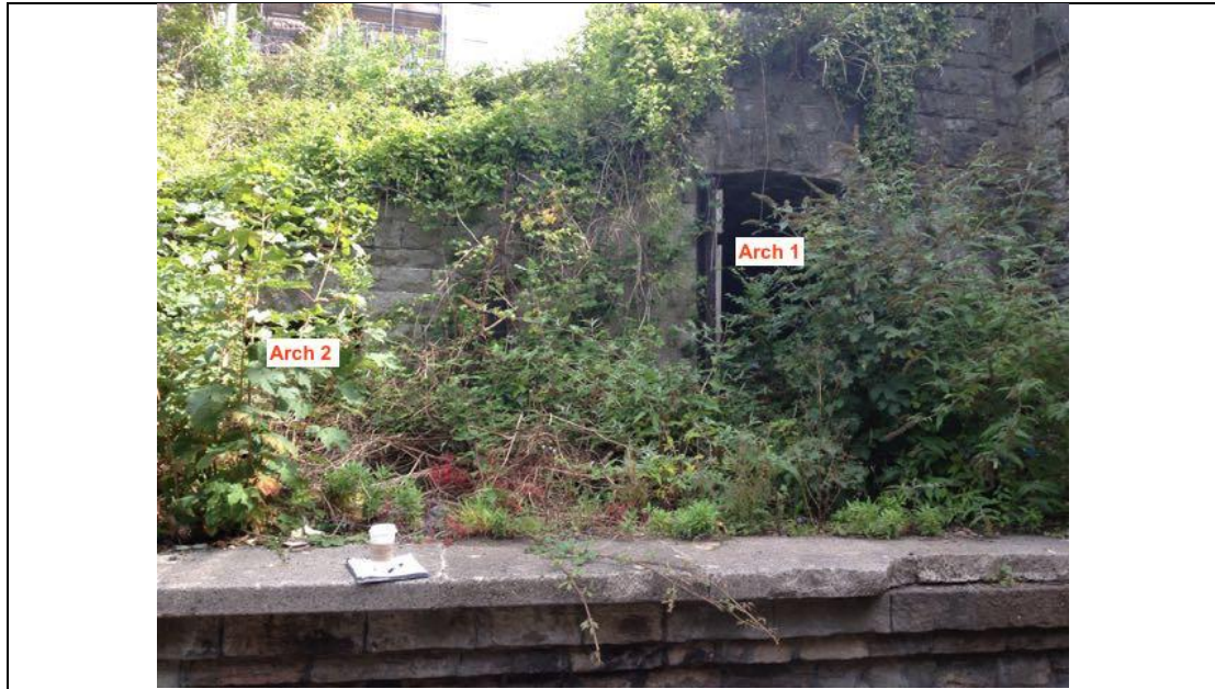
Plate 1. Arches on Pill Station Platform
