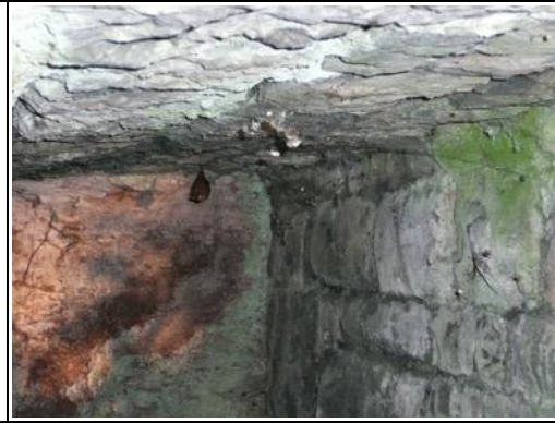
Photo 18. Bat roost at Pill Station Arch (Lesser horseshoe bat) Date: September 2016
